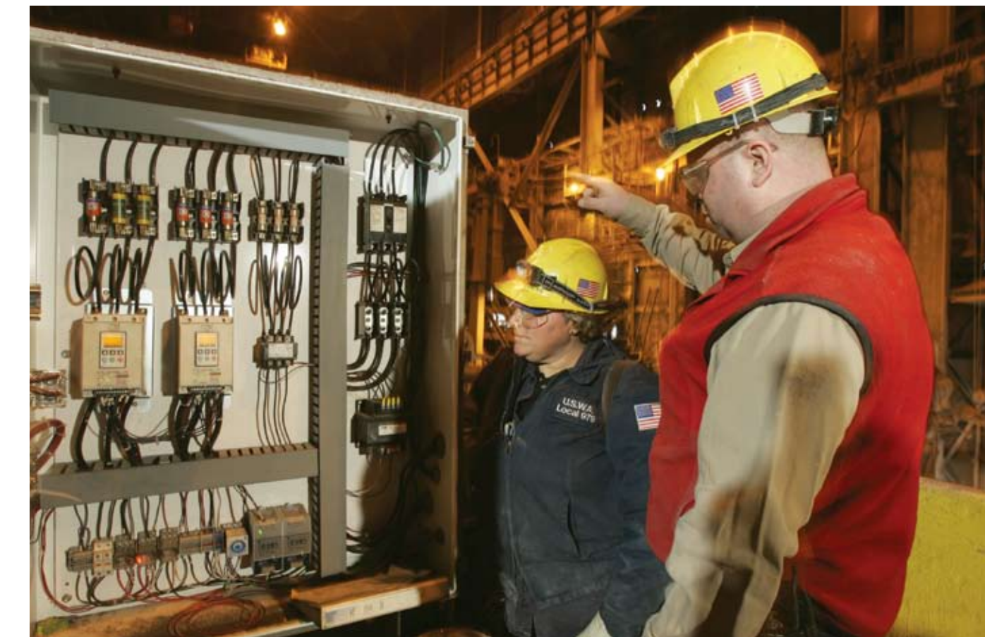
An employee at ArcelorMittal-Cleveland prepares for Maintenance Technician-Electrical certification.
