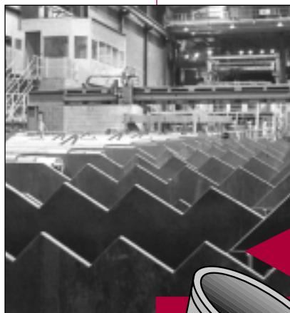
New cooling racks for steel bars have been installed at CSC Ltd. as part of the company's modernization project.
