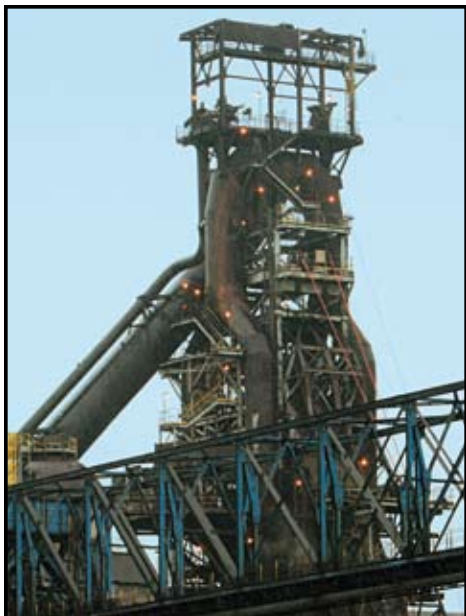
Gases from blast furnaces such as this one at ArcelorMittal Cleveland are captured and recycled to produce electricity.
